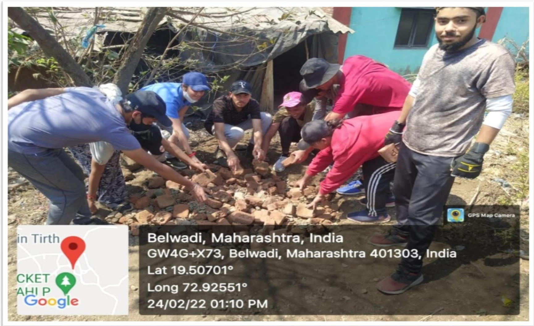
Soak Pit Making at Belvadi 22 nd to 28 th February 2022
